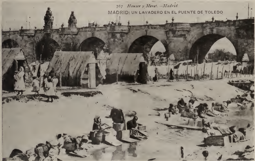
BRIDGE, AND A WASHING PLACE BY THE RIVER, MADRID
